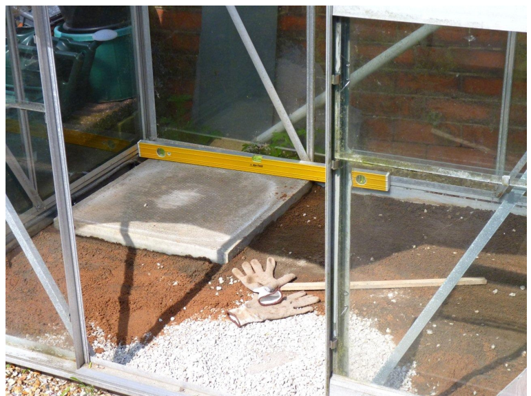
Floor levelled and first paving slab in place
